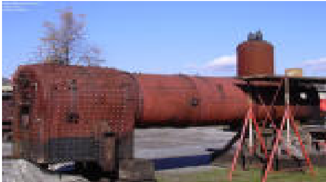
Old Locomotive Boiler
