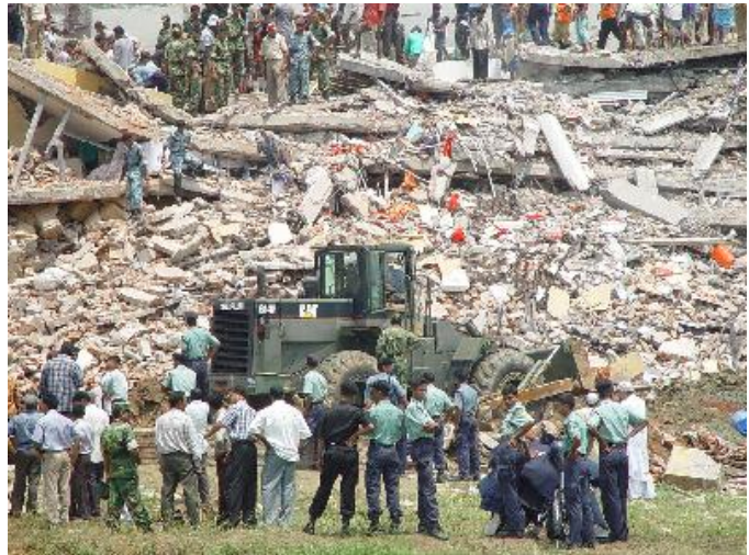
12 killed in Bangladesh Boiler Explosion
